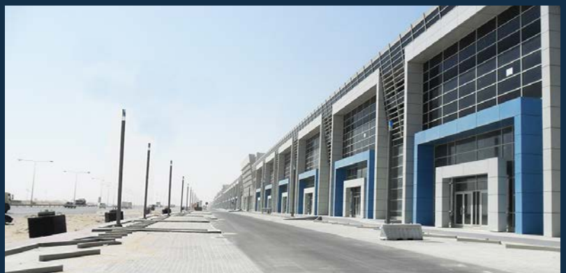
Road Works for Barwa Commercial Avenue.
