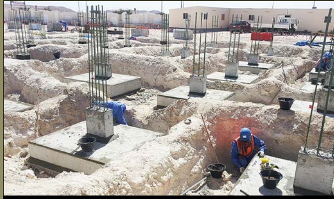
Dukhan Housing Project Phase 9
